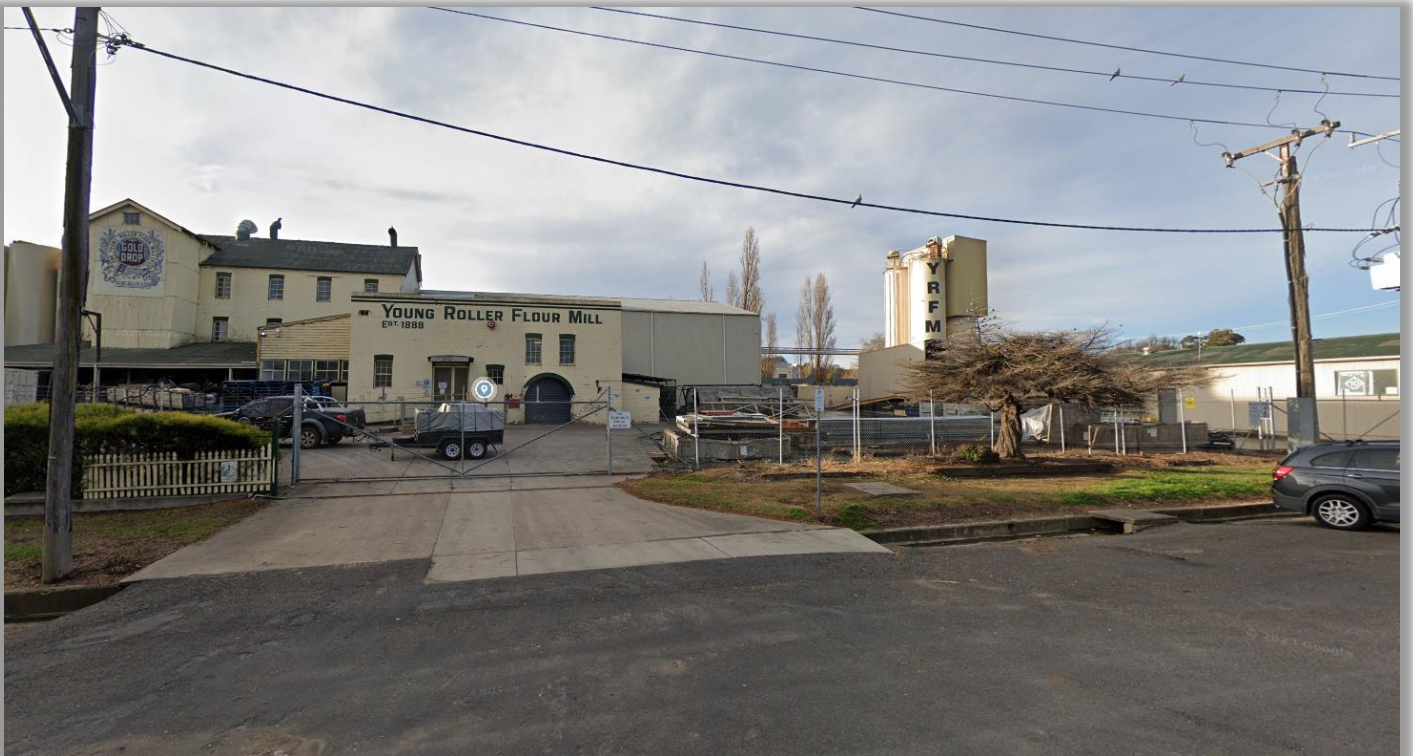
Historical Flour Mill buildings to left – site of new extension to right.
