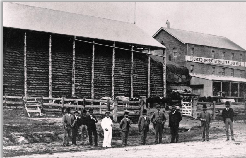
Estimated age of image late 1890's – note storage shed & original mill building Source: Dr R Longdin – Monitor Heritage Services 2014
